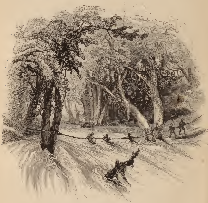
RUDE BRIDGE OVER THE OVIGUI.
